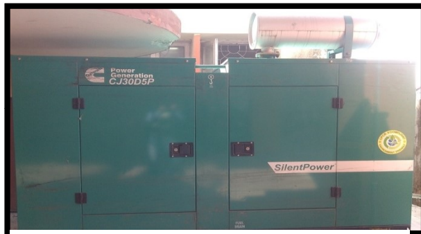
GEN SET AT DATA CENTRE, DUDH
