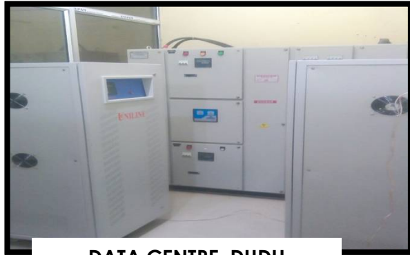
DATA CENTRE, DUDH
